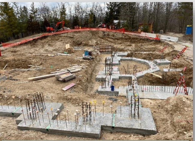
3.30.2020 - Foundations of the New Chapel
