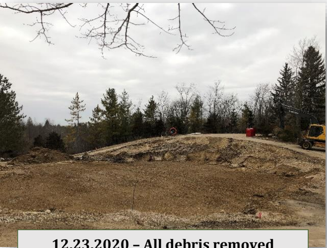
12.23.2020 - All debris removed
